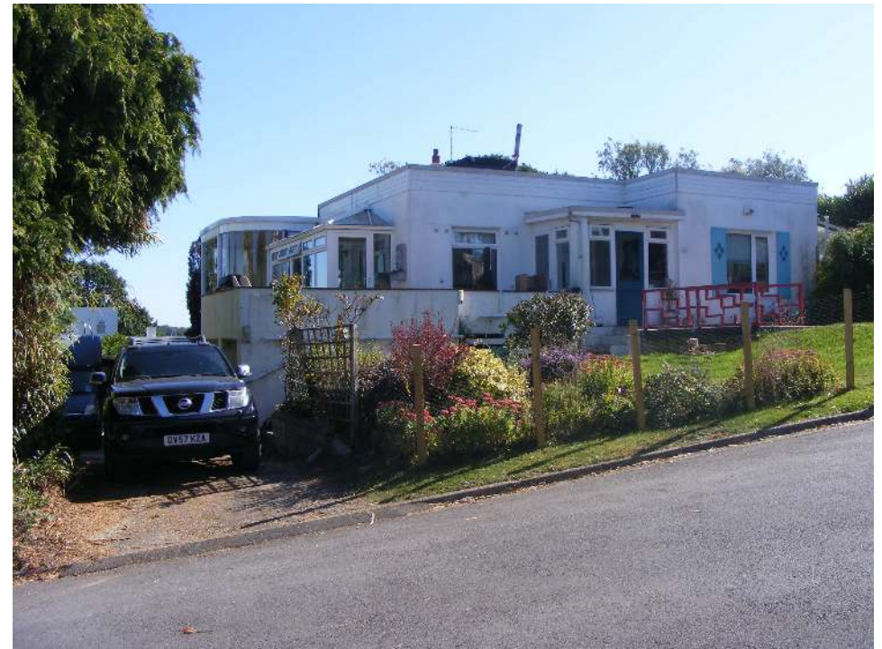
(02) Photo looking South-East at No.14A Crowsport Estate from the level of the front access drive, highlighting the properties mass, material character, site topography and existing nature of the front garden with associated boundary treatment.
