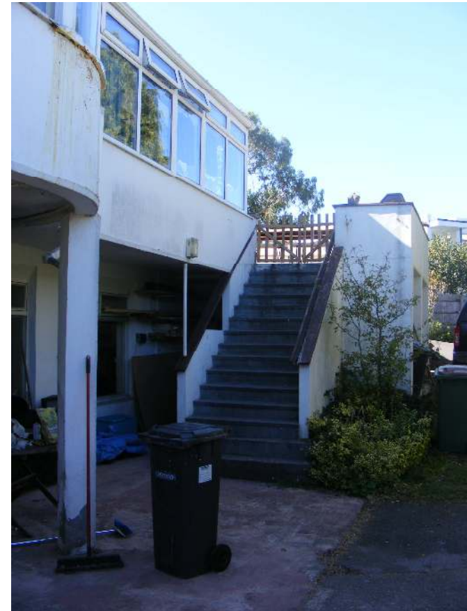
(04) Photo looking west highlighting the overall mass, material character and changes in level between the lower car parking area and the upper ground floor terrace. In addition the photo also highlights the extent of the existing North facing conservatory and weathering issues associated with the projecting curved bay window.
