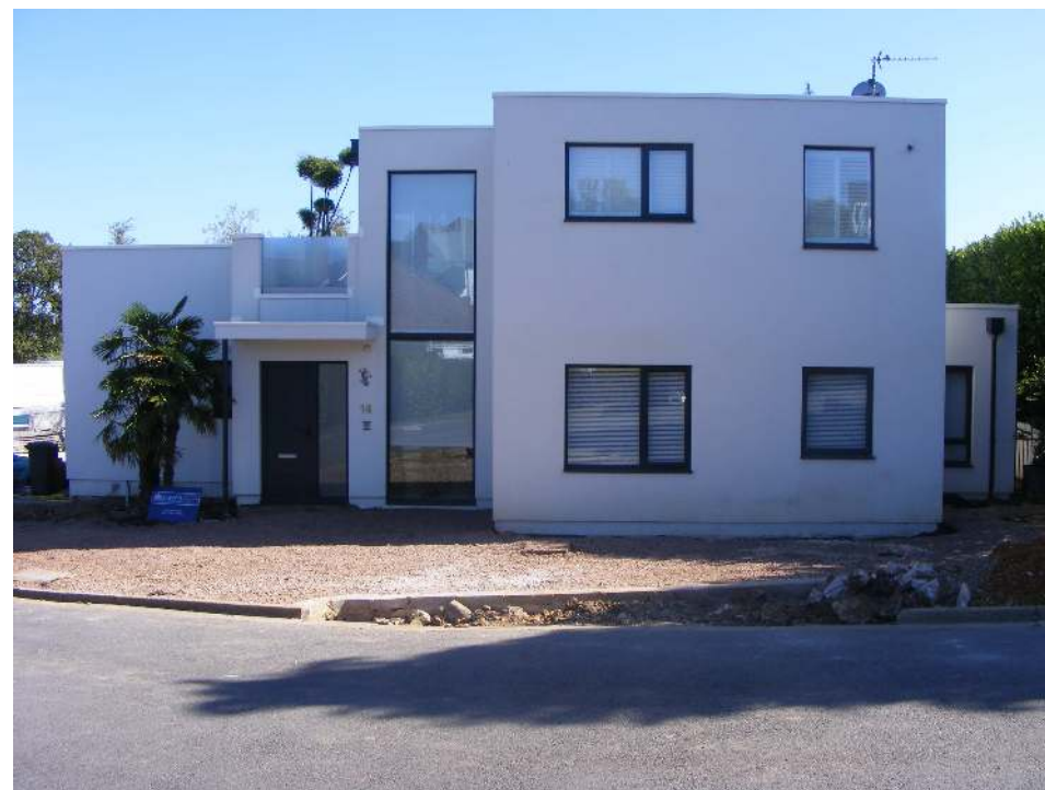
(08) Photo of No.14 Crowsport Estate, recently extended and remodelled to include new first floor accommodation and an associated roof terrace, as per Planning Approval C/15/76351 (details confirmed in Appendix A).
