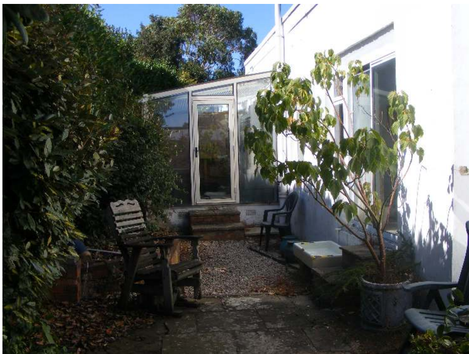
(07) Photo looking West along the raised rear patio / terrace area, highlighting the character of the existing rear conservatory, proposed to be replaced with a new utility room, maintaining access to this area
